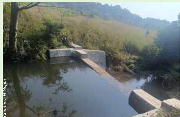
Check dam to channel water in Kuls
